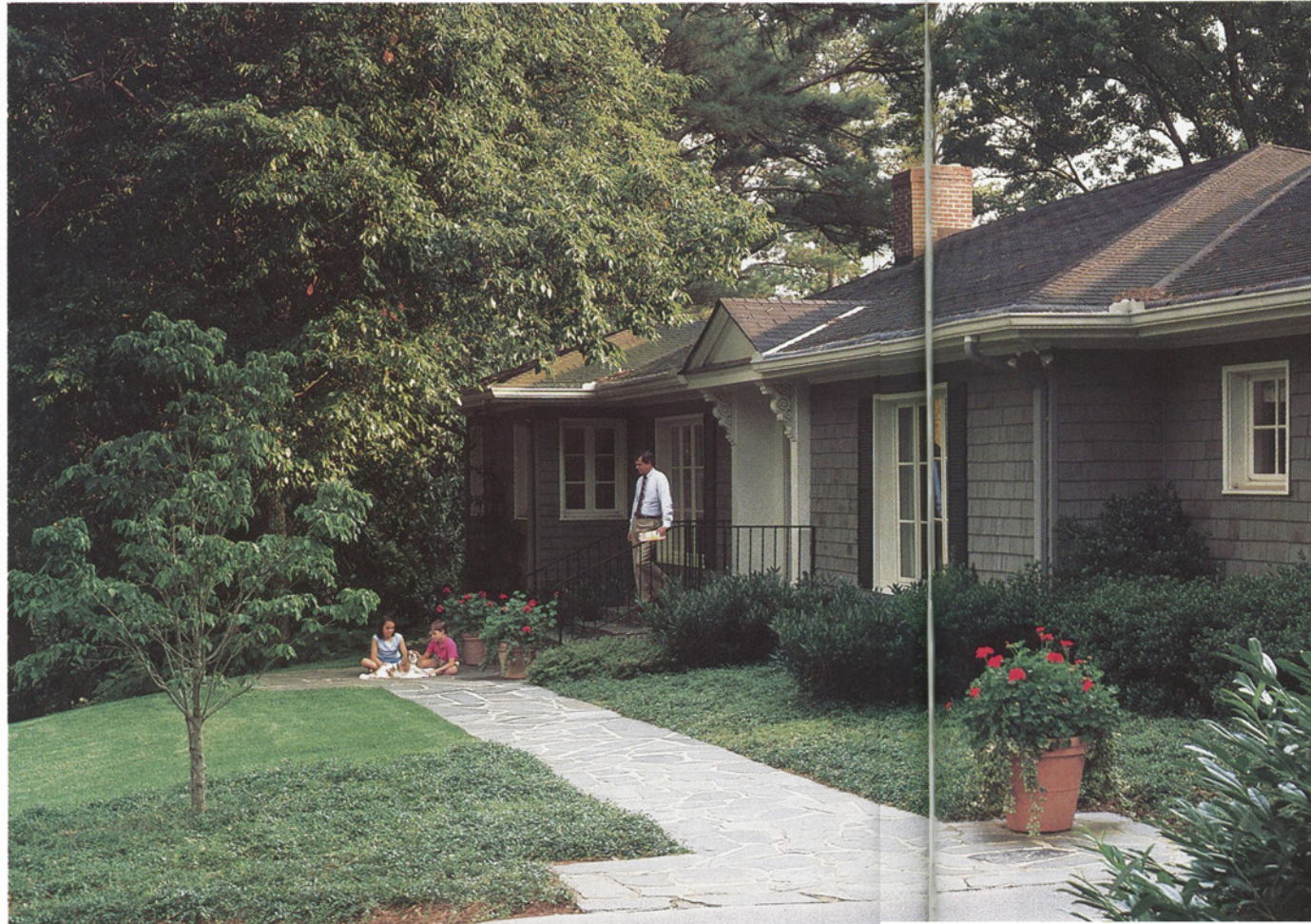
(Above) Cindy and Bobby Candler's Atlanta home has a fresh new look. (Right) Before renovation, the sloping lot, brick facade, and metal windows made the house typical of those built in the fifties. (Bottom, right) Changing the entry so you approach the steps from the front rather than the side made it more appealing. Photographs: Van Chaplin
